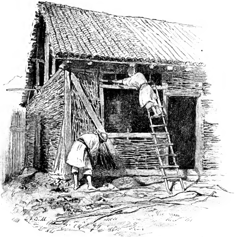
BUILDING A HOUSE IN SERVIA
